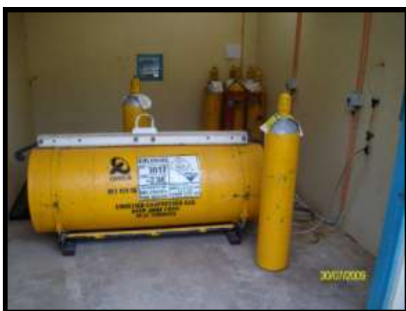
Gas chlorine cylinders -920 kg
