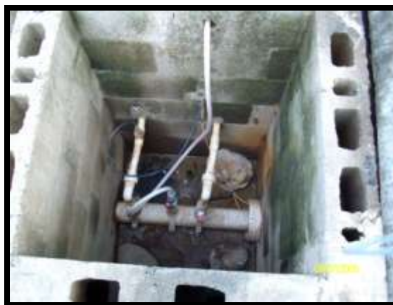
Chlorine drip injection -Qereqere
