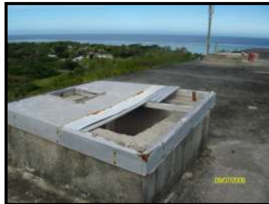
Voua Reservoir – Damaged lids
