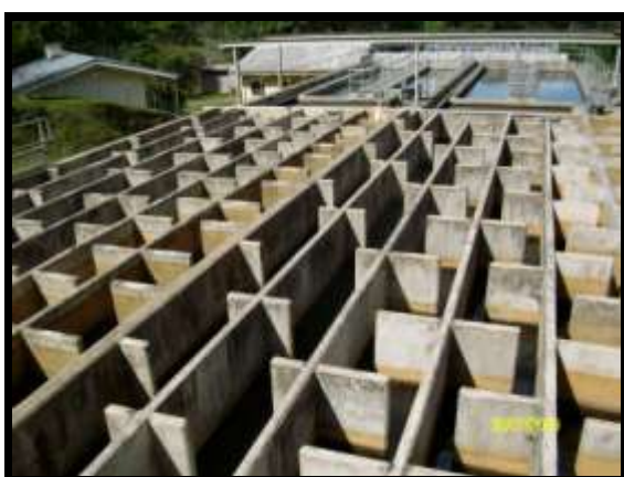
Horizontal clarifiers and Sedimentation Tanks
