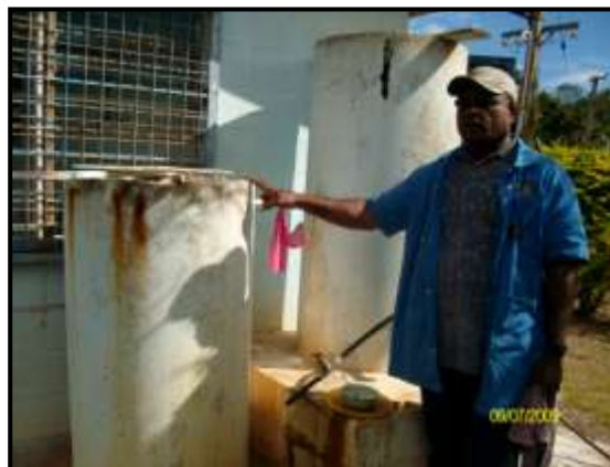
Manual Chlorination-Qereqere Pump Station
