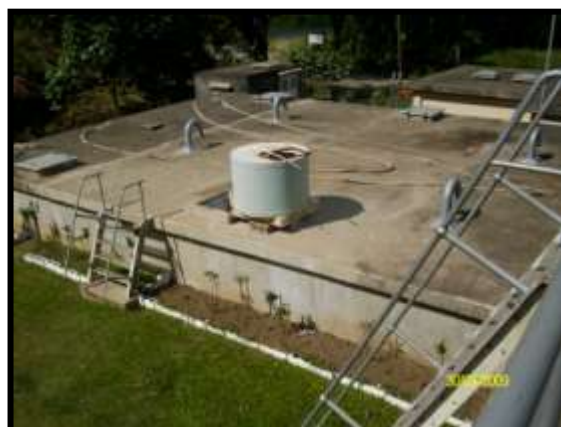
Manual Chlorination Tank on Contact Tank 1
