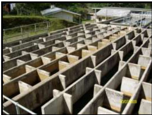
Horizontal - Maze Clarifier – Matovo Plant
