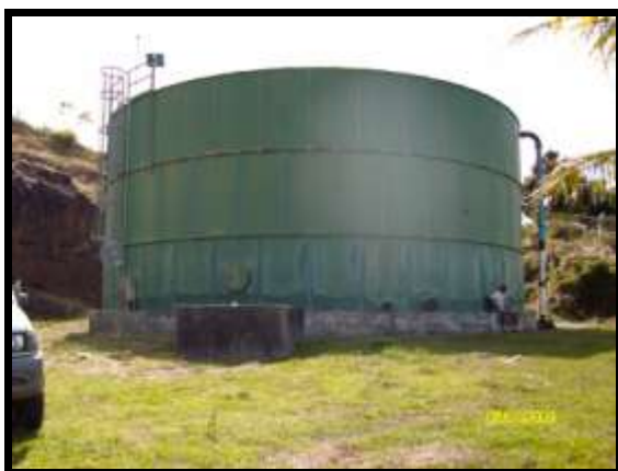
Lawai Reservoir – New -Steel Bolted
