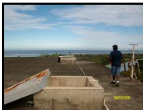
Voua Reservoir – Damaged lids
