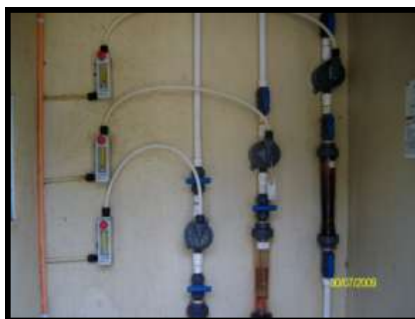
Functioning Chlorinator
