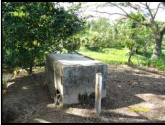
Borehole Intake at Qereqere - Sigatoka
